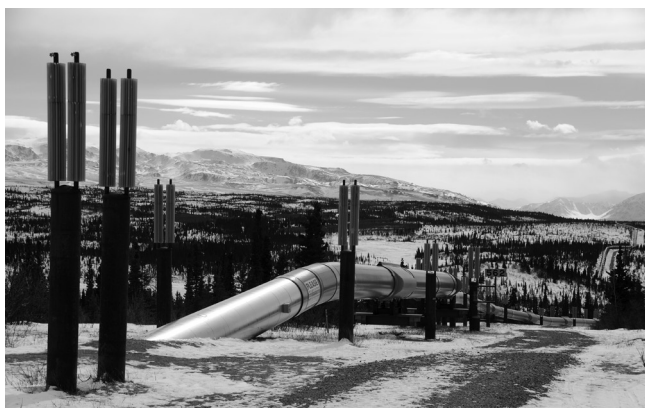
Oil pipeline in the Tundra
