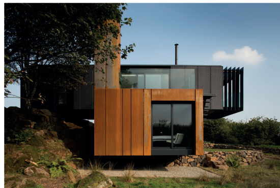
Grillagh Water House , Northern Ireland (2014) by Patrick Bradley Architects Materials: recycled steel shipping containers, glass, colour coated metal, pre-rusted steel cladding
